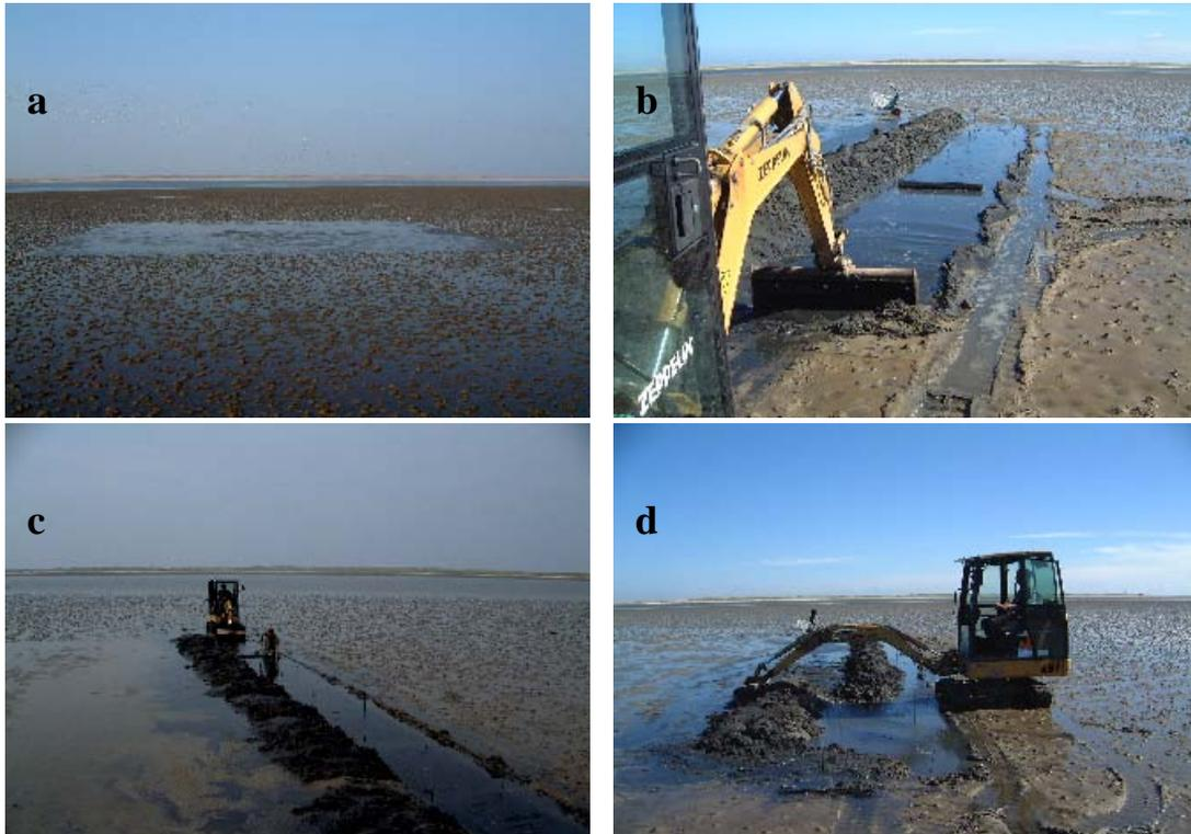
Fig. 3. Creating of lugworm exclusion plots (a) was achieved by excavating the upper 10 cm of the sediment with a small backhoe (b) and inserting a 1mm meshed polyethylene net (c) before returning the sediment (d).
